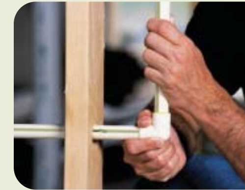
AMONG THE MANY ADVANTAGES OF EVERTUFF IS EASY, PERMANENT JOINTING USING SOLVENT-WELDED CEMENT FUSING.
