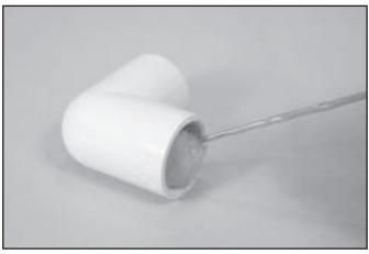
Apply a medium coat to the fitting socket. Avoid getting cement in other sockets or threaded connections.
