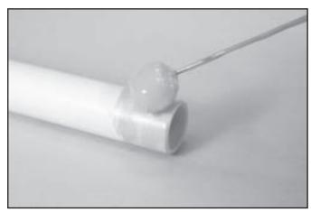
Apply a heavy, even coat of cement to the outside of the tube end. Work the cement into the joining surfaces using a continuous, circular motion.
