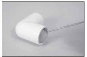
Apply a medium coat to the fitting socket. Avoid getting cement in other sockets or threaded connections.
